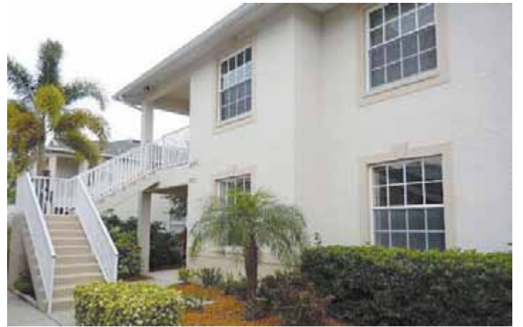
1001 AUBURN LAKE CIRCLE #1, VENICE, FL 34292 - 2 bed 2 bath ground floor condo! Cozy interior features ceiling fans, a breakfast nook and a screened-in patio that overlooks the large lake in the back. Easy access to I-75. Located close to Venice beaches. There is also a community pool and spa, clubhouse and gym. $179,900. Call Anytime Realty LLC (941) 276-9290 PDR812 Ad Code: FM2316372
